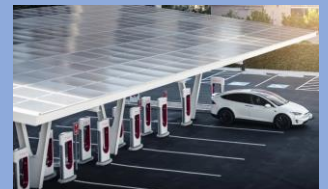
A Solar EV Charging Station
