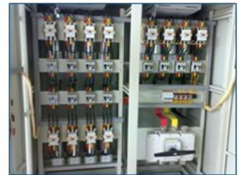
**Capacitors:** Many large users of electricity are charged for something called "Power Factor". If the Power Factor is less than 90%, then they are wasting electricity. A Capacitor Bank corrects this, and makes the power supply far more efficient and cost effective.
